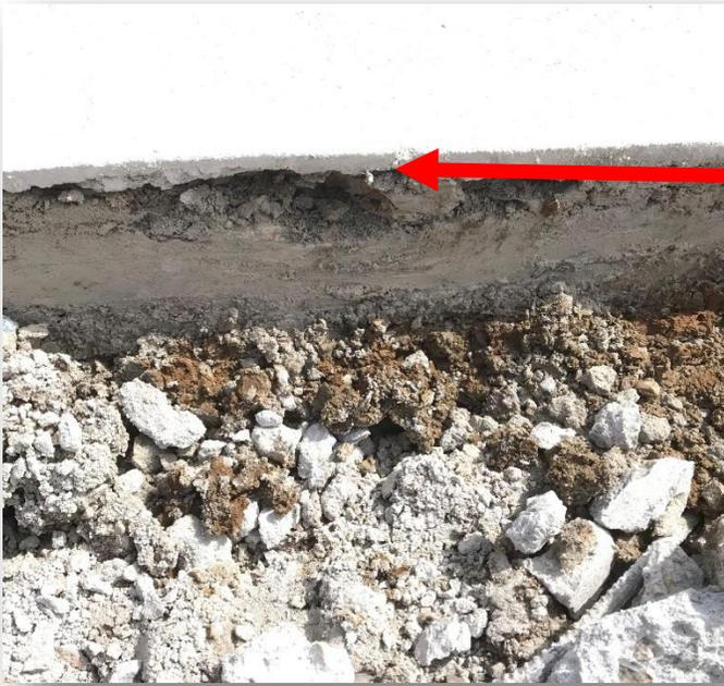
The Concrete has broken down over the past two decades and, in some areas, remaining was less than 1 inch thick, resulting in cracks and spalding
