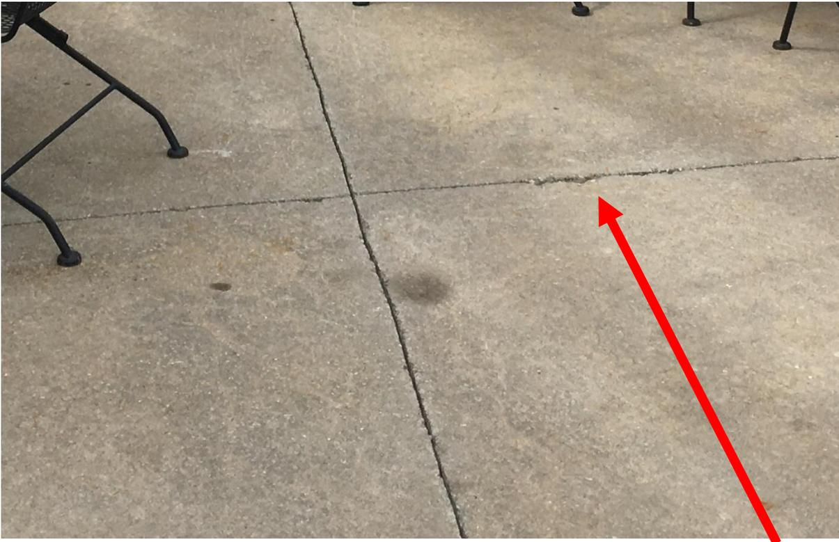
Parts of slabs crumbling and many small and medium cracks allowing water to cause further damage
